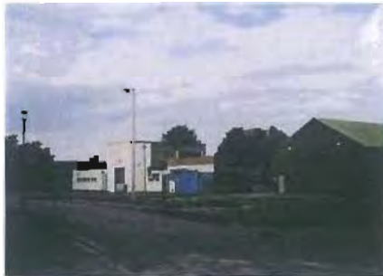
Re-Use of Buildings on Redundant Air Bases
