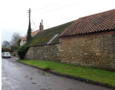
Figure 21 Limestone walling and pantile roofs of barns on the east side of the "Wetherwalk".
