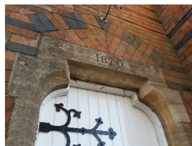
Figure 28 Red and blue brick and stone detailing of the village hall.
