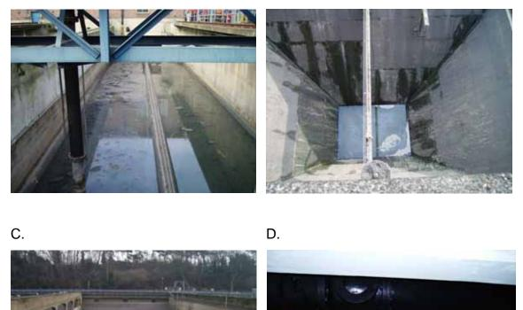
Fig 10. Mosquito breeding sites at Mogden STW, London. Stationary grit removal channels (A) and the sumps (B) of the storm tanks (C) can all provide larval breeding sites. The areas beneath the aeration tanks (D) can provide adult overwintering sites and, where leaks occur, intermittent larval breeding sites. These potential breeding sites are common to many STWs.
