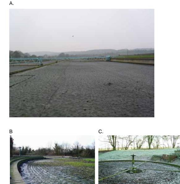
Figure 1. (A.) The filter bed at Esholt STW (West Yorkshire) showing one of the 52 acres of filter bed present at this site. (B) A typical medium sized plant at Marehay, Derbyshire, consisting of four filter beds. (C) A small STW at Huggate, East Yorkshire, consisting of two small filter beds and serving a village of approx. 500 inhabitants.
