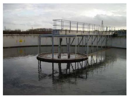
Fig. 2. The activated sludge process at Derby STW (a modern five year-old plant that replaced a large filter bed facility). Aeration ponds (A) comprise of constantly moving sewage that do not allow for the breeding of insects. Similarly, the final settlement ponds (B) have never given rise to insect problems. The surrounding area, where filter beds had previously been present, provided no obvious breeding sites for aquatic insects.
