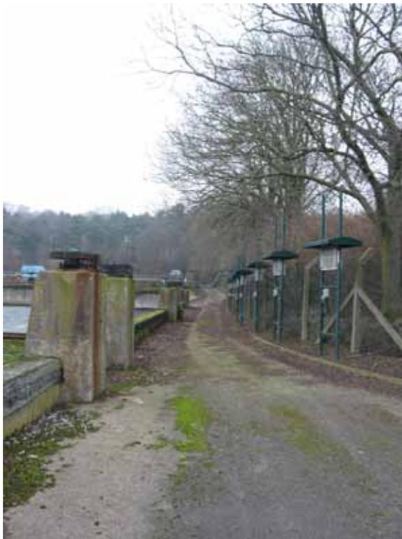
Fig 9. (A) The filter bed matrix typically comprises of stones over which the zoogloea growth forms. Egression of flies in problematic filters is frequently prevented by enclosing the entire filter with netting (B). The netting becomes efficient only when the zoogloea growth permeates the perforations in the net. UV/electrical killing grids located downwind of the filter beds at Esholt STW, West Yorkshire.
