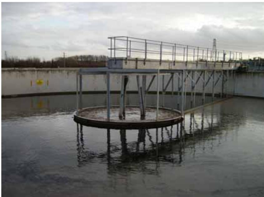
Fig. 2. The activated sludge process at Derby STW (a modern five year-old plant that replaced a large filter bed facility). Aeration ponds (A) comprise of constantly moving sewage that do not allow for the breeding of insects. Similarly, the final settlement ponds (B) have never given rise to insect problems. The surrounding area, where filter beds had previously been present, provided no obvious breeding sites for aquatic insects.
